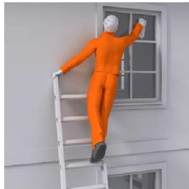
✗ Figure 3 Incorrect – overreaching and not maintaining three points of contact (means of securing omitted for clarity)
